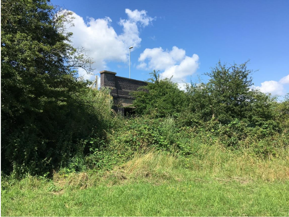
Looking north west at north western corner
